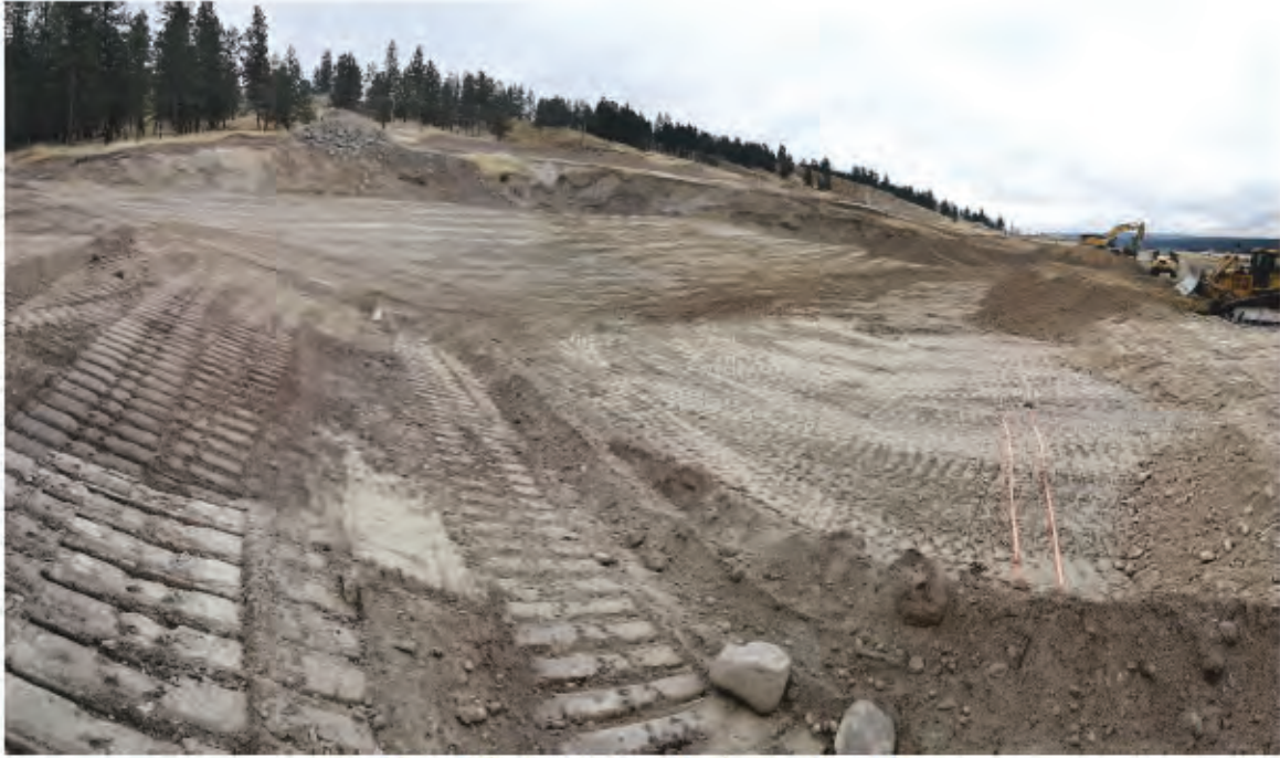
Figure 1 Finished slope and beginning of new lift
