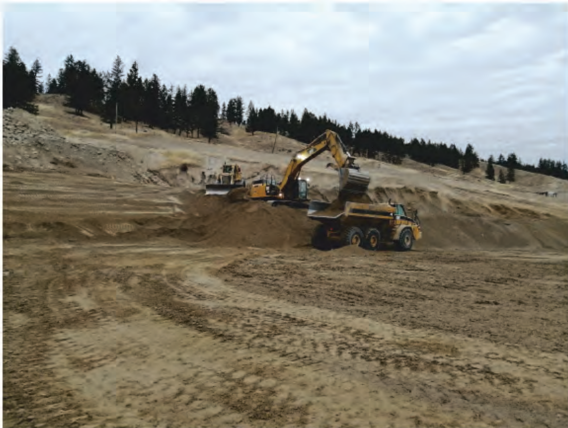
Figure 2 Progress of excavation and slope construction
