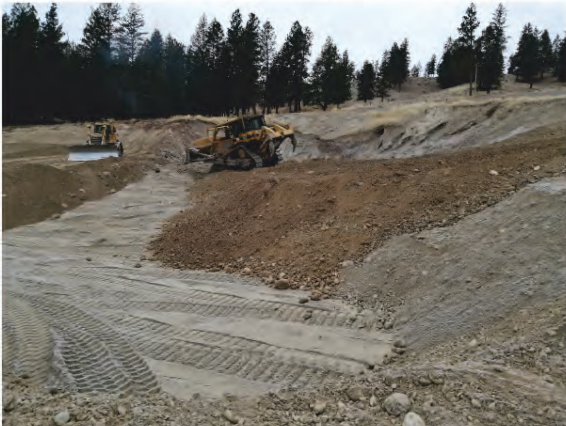
Figure 2 Slope shaping example
