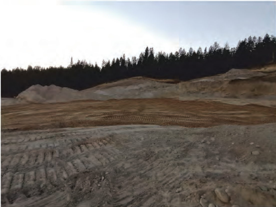
Figure 2 Initial lift after placement
