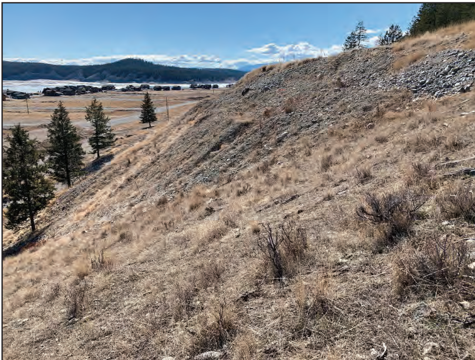
Photo 8: Looking southerly along east-facing slopes between southern and northern areas. Note transition from natural slope (in foreground) to oversteepened granular fill slope in distance (March 16, 2021).
