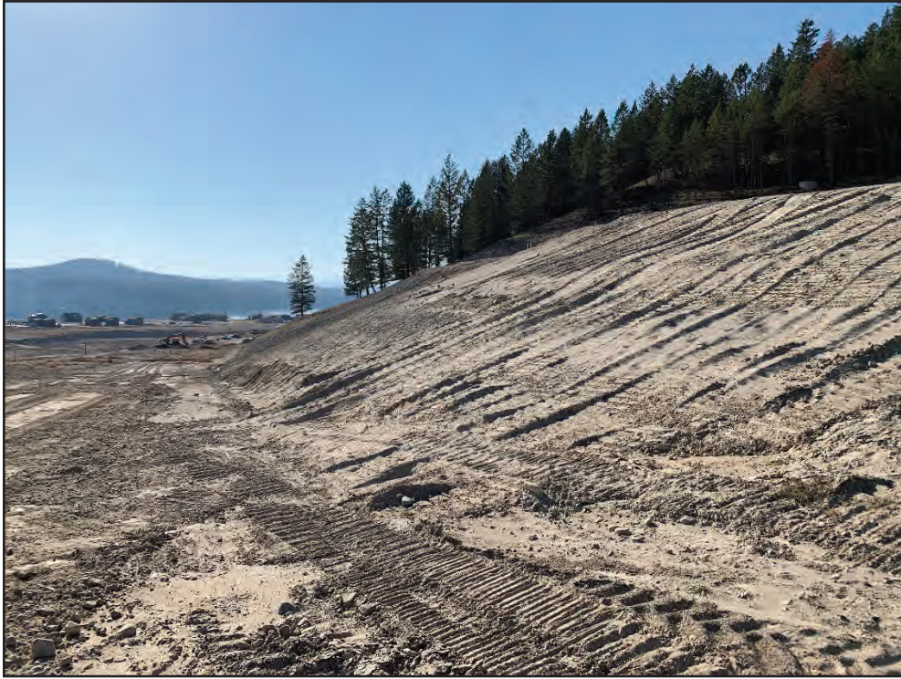
Photo 13: Middle Terrace Phase 2. Profile view of graded east-facing slope on Lots 77 and 78, looking southerly. Surficial silts and sands were encountered in this area (October 19, 2021).
