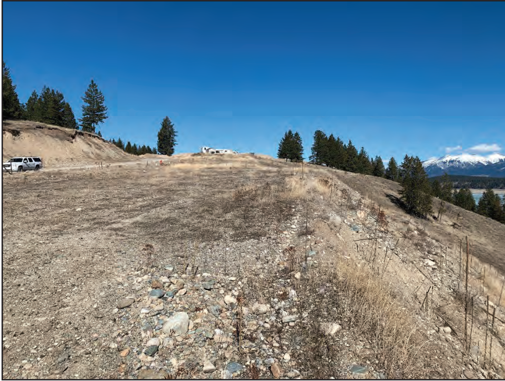
Photo 9: Middle Terrace Phase 2. Looking north along crest of east-facing slope between southern and northern areas (March 16, 2021).
