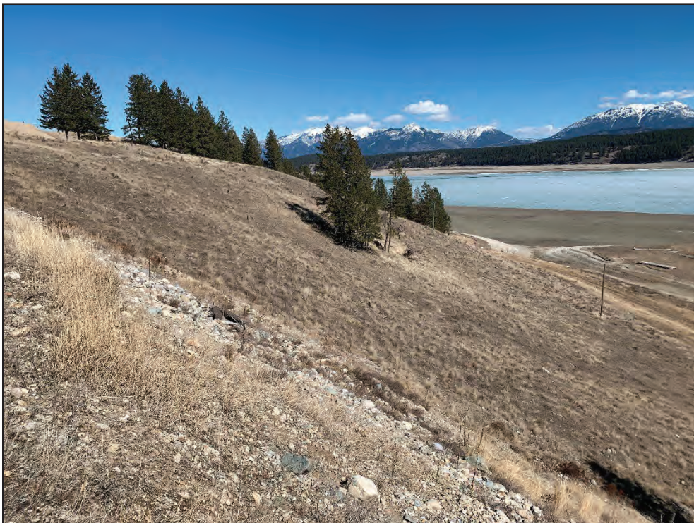
Photo 10: Profile view of undisturbed (grass-covered) southeast-facing slope on Lots 74 to 76 in northern area. Oversteepened granular fill slope can be seen in foreground (March 16, 2021).
