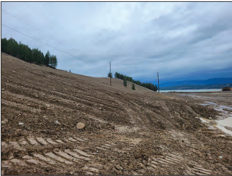
Photo 16: Profile view of east-facing slopes in southern area following buttressing/dressing. Photo by E. Mueller (November 30, 2021).
