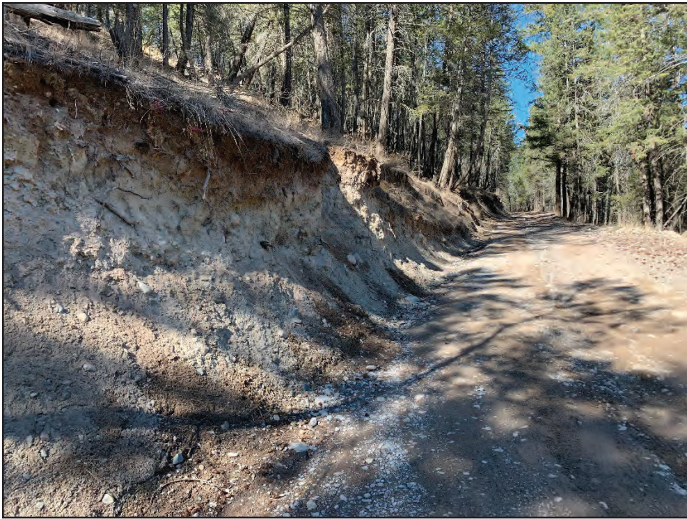
Photo 14: Profile view of steep road cut along rear (southwestern) boundary of Lot 82. Material exposed is glacial till (March 16, 2021)
