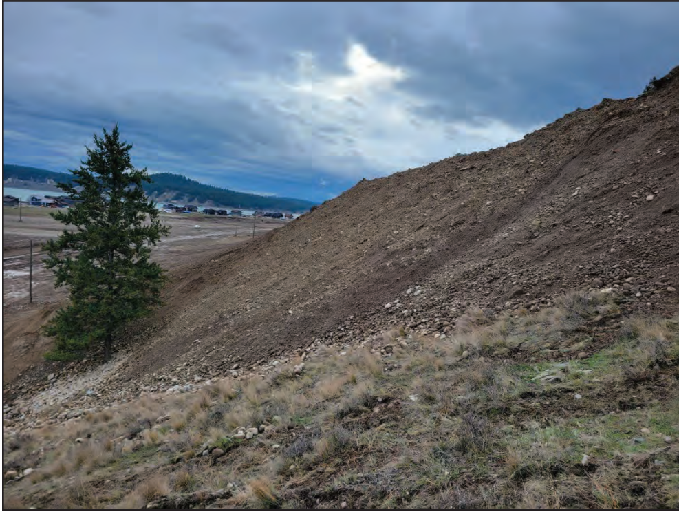
Photo 17: Middle Terrace Phase 2. Looking southward at buttressed/dressed east-facing slopes between southern and northern areas. Photo by E. Mueller (November 30, 2021).
